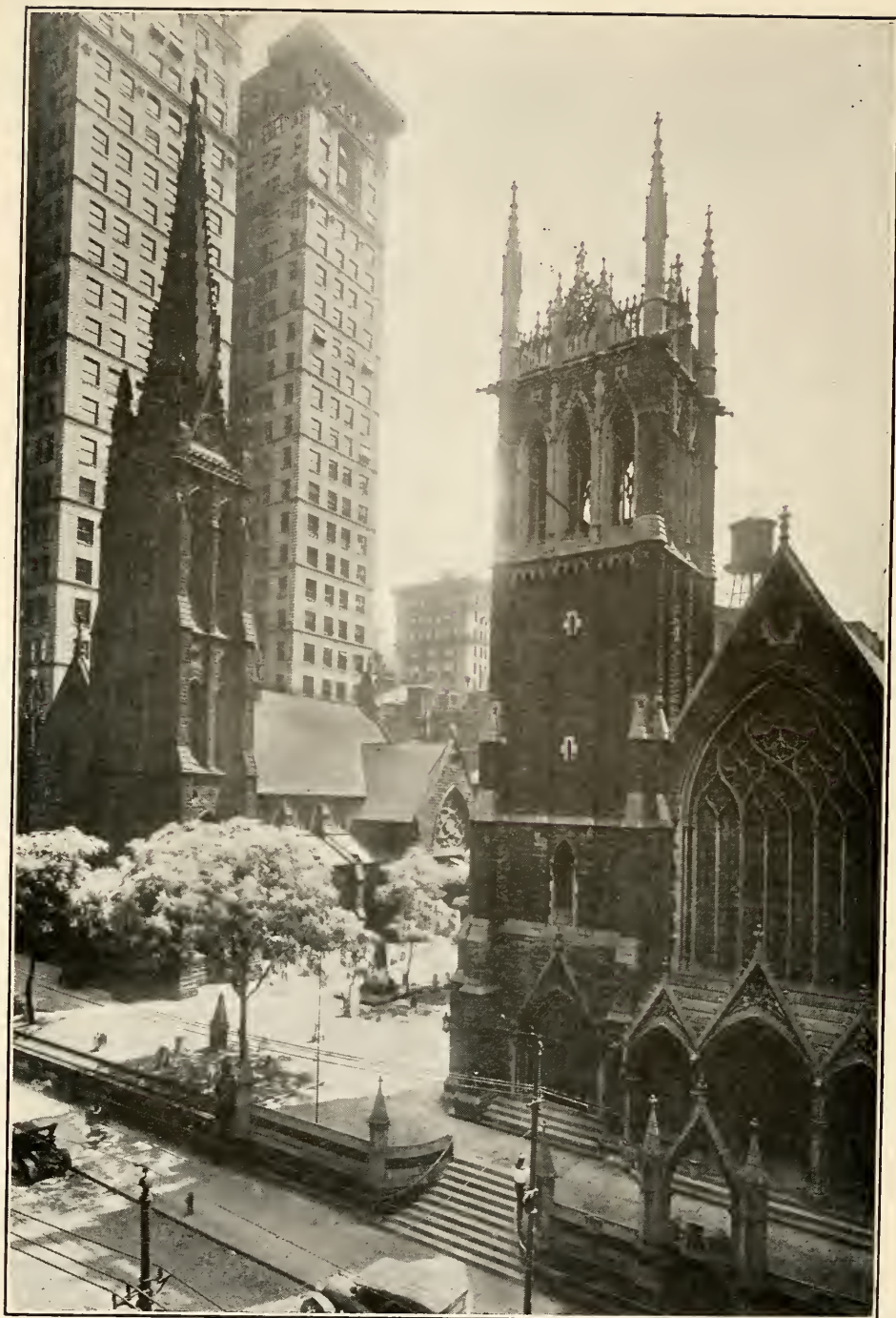
Trinity Court Studio, R. W. Johnston. First Presbyterian Church and Trinity Church Today. Oliver Building on the left.
